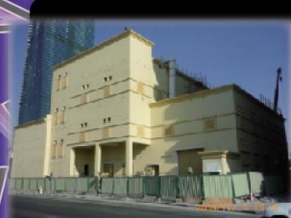
Main Building of Trade Centre Roundabout (North-Eastern View) Substation in Dubai
